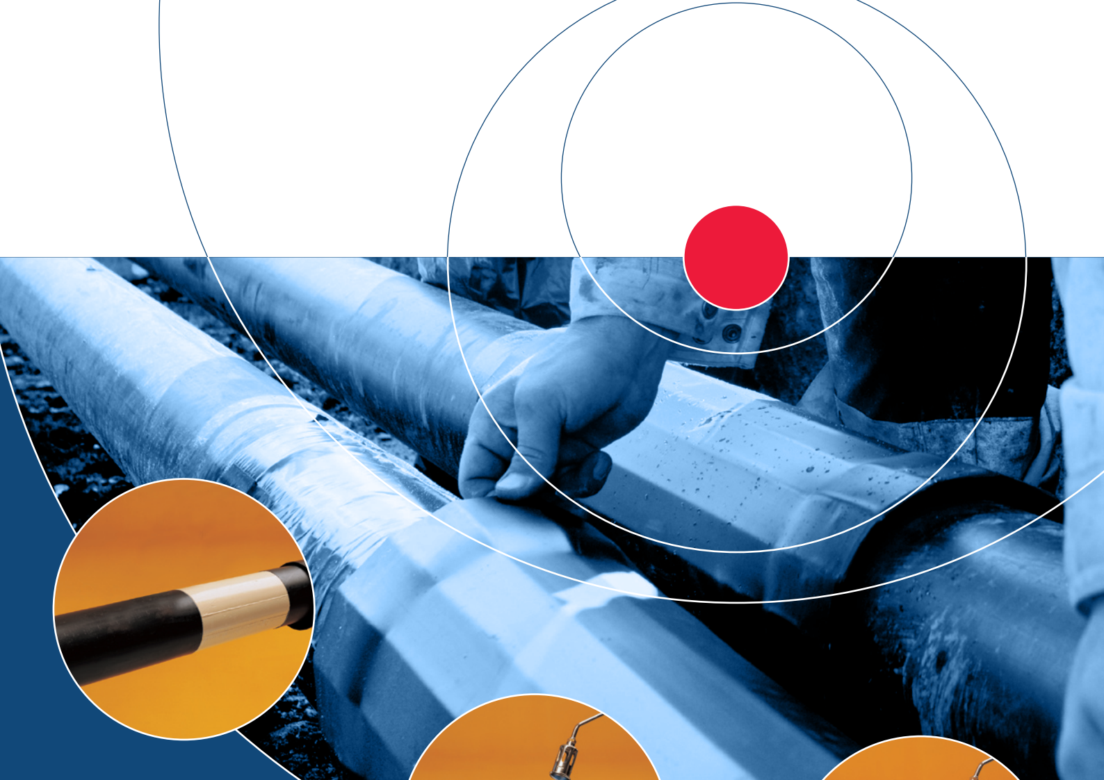
Adjusting the insulation sections
