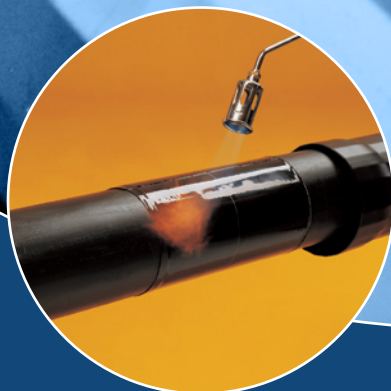
Shrinking the shrink foil First seal
