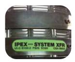
MJ Grey couplings can be easily differentiated from standard cast iron couplings by noting that the rubber interior sleeve is grey in colour (versus the traditional black colour) and exterior identification labels showing the System XFR trade name and the Flame and Smoke values as per ULC S102.2.
