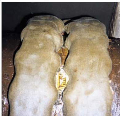
Denstyl Mastic Blankets applied to flange pair.
