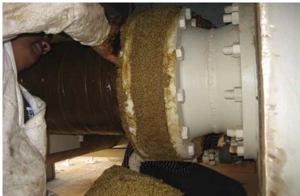
Denso Profiling Mastic will adhere to metal, PVC, polyethylene and concrete.
