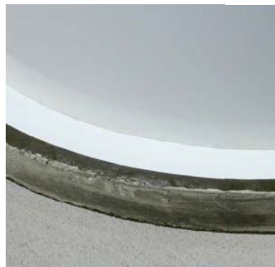
Denstyl Mastic applied to protect tank bases from corrosion.
