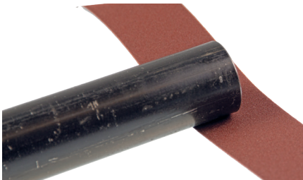
FIGURE 9: CLEANING PIPE
