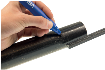
FIGURE 8: MARKING INSERTION DEPTH
